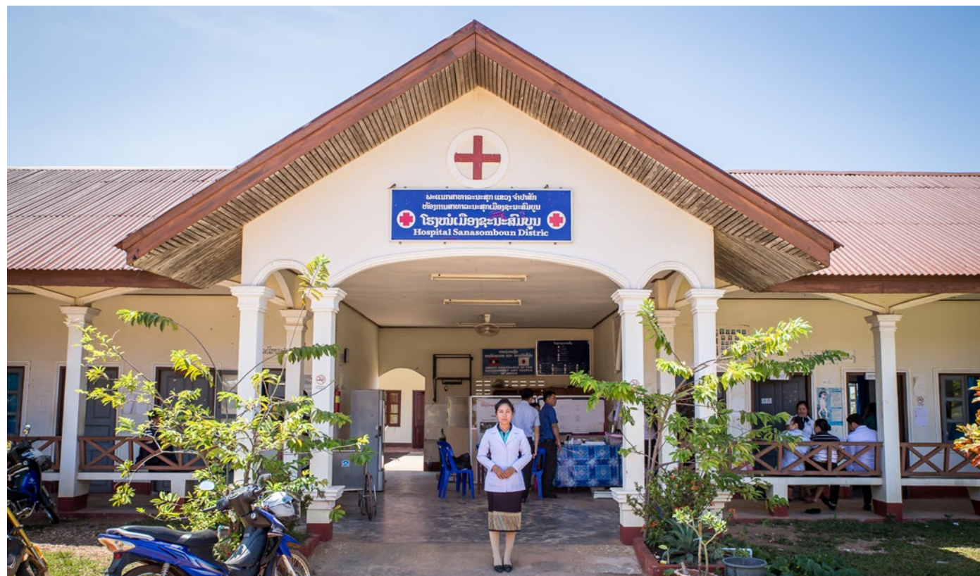
THE SANASOMBOUN DISTRICT HOSPITAL LAO PDR
